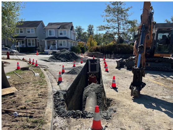
Water main construction in South Surrey
