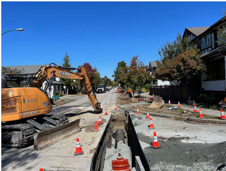
Engineering team on watermain construction site in Surrey
