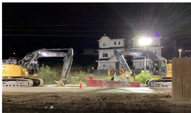
Construction of 16th Avenue Trunk Sewer at 168th Street
