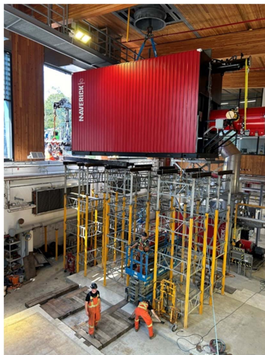
New Boiler Being Lowered into West Village Energy Centre
