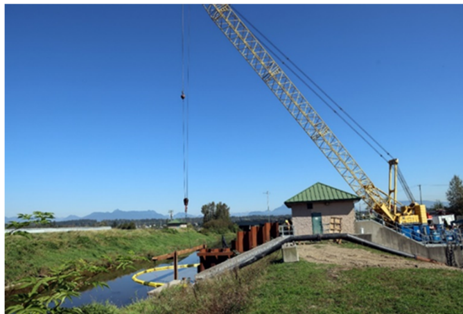
Sheet pile installation at the Fry's Corner Pump Station
